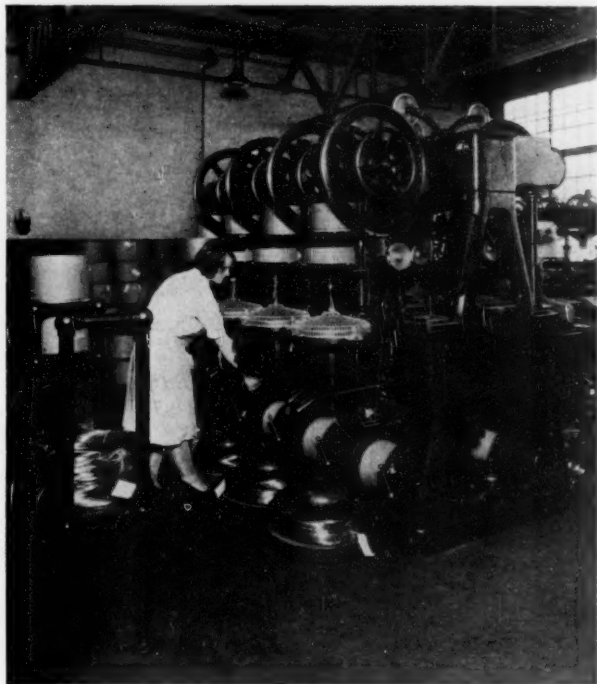
Fig. 6—Paper insulating machine.
