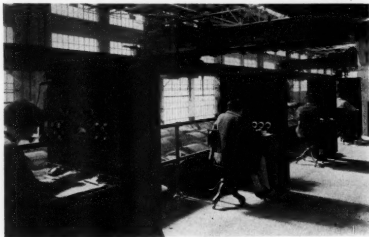
Fig. 30—Typical test set installation at Baltimore plant.
